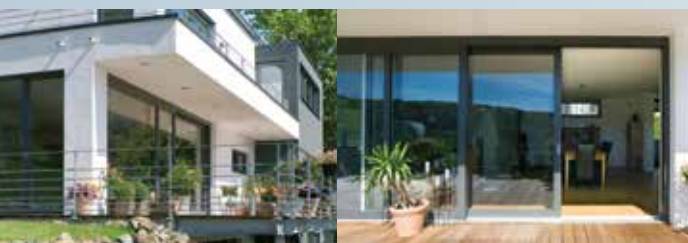
One lift/sliding sash and one fixed pane
